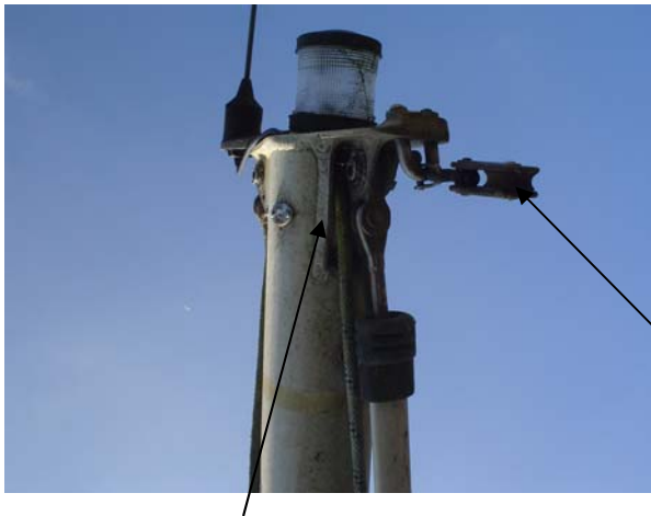
Remove and inspect sheave
