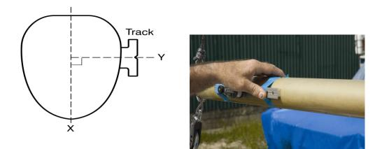
Remove track, drill using 4.2mm drill and tap using 5mm tap then secure in position using 5mm machine screw
